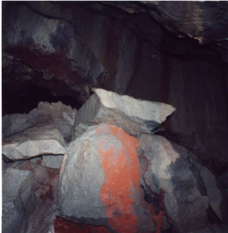
Fig. 10 - Botte dell'Acqua (water barrel) Quarry; example of vault collapse: this phenomenon is widespread throughout the quarry and often stops up the passage. A lava-stone slab in contact with the « agghiàra » and traces of water dripping through the vault cracks can be observed (pict. by R. Bonaccorso).
