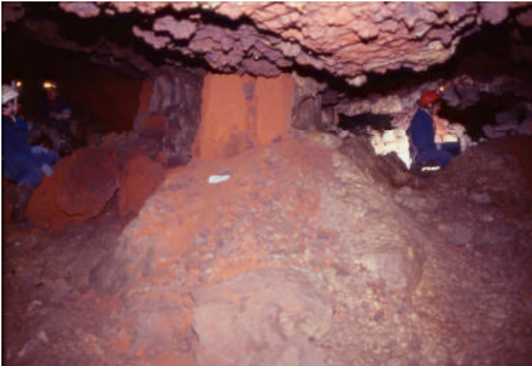
Fig. 8 - Botte dell'Acqua (water barrel) Quarry; residual «agghiàra» pillar close to material partially collapsed from walls and vault (pict. by A. Marino).
