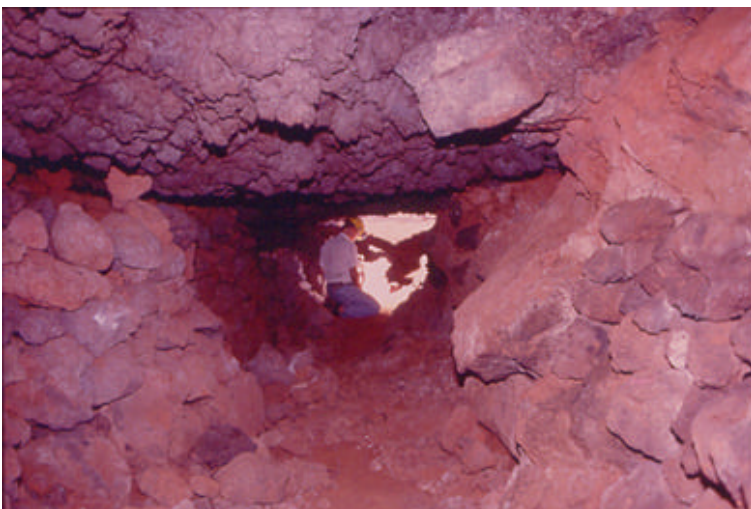
Fig. 8 - Botte dell'Acqua (water barrel) Quarry; residual «agghiàra» pillar close to material partially collapsed from walls and vault (pict. by A. Marino).
